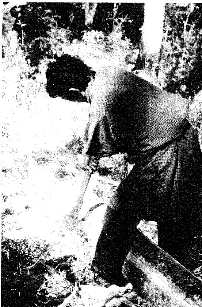
Figure 6-2: Processing of a beam, below the village of Dhur, 1997.
