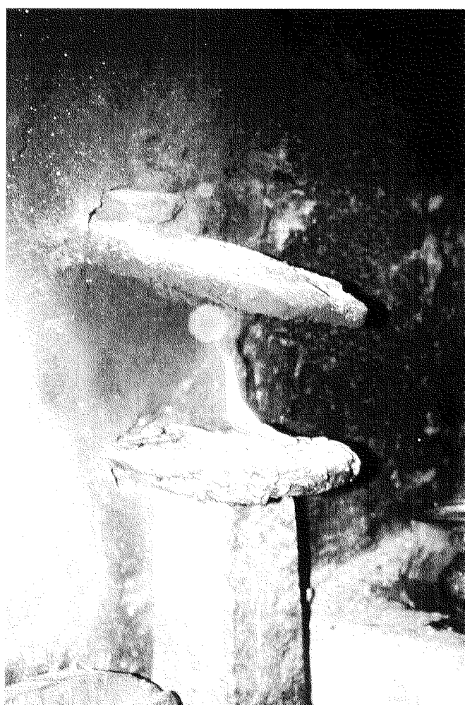
Figure 6-7: A “ kuan holder” in a old house in Dhur. The kuan is laid on the lower stone. The soot is collected on the upper stone. Dhur, 1996.
