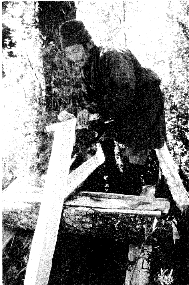
Figure 6-5: Processing of shingles, Dhur, 1997.
